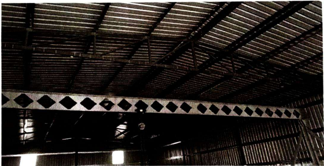
Fig: - Roof Truss. (Field House)
